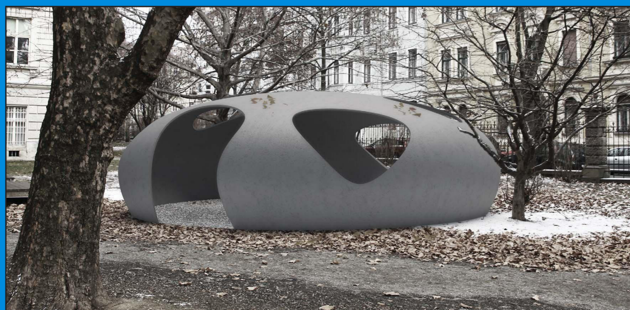
UHPC learning pavilion at the campus of the TU Graz – student work by Stephanie Jordan, Nikolaus Pfusterschmied and Felix Zmölning
