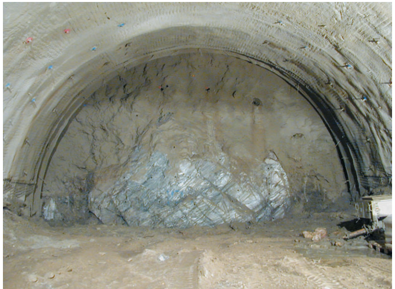
Fig. 3 Large boulder of quartz-phyllite encountered at station 161 m.
