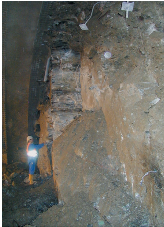
Fig. 4 Bedrock contact at station 191 to 192 m.
