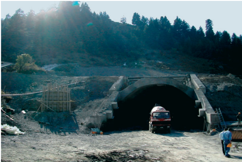
Fig. 3 East portal of the Anilio Tunnel.
