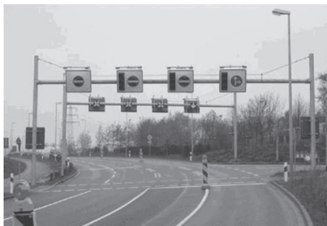
Figure 14. Urban contraflow system next to Nordpark Mönchengladbach. (Reproduced with permission from Grimm GmbH.)
