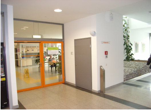
Fig. 3. (right): The position of the Exiter within the building
