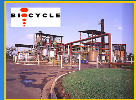
Industrial plant for PHA production (here: PHBISA, Brazil)
