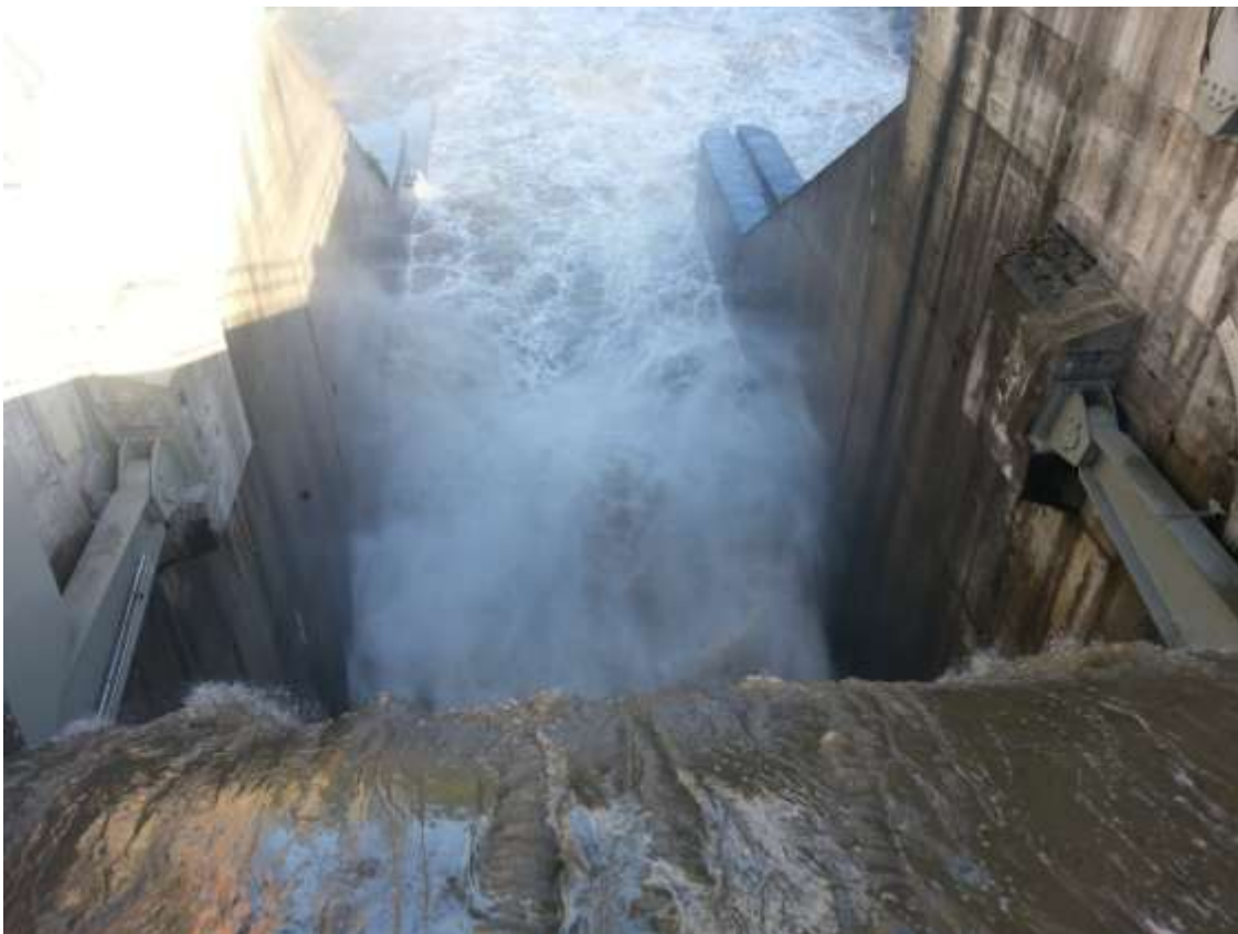
Figure 1: Hydropower plant Bodendorf during a flushing of the reservoir in July 2012
