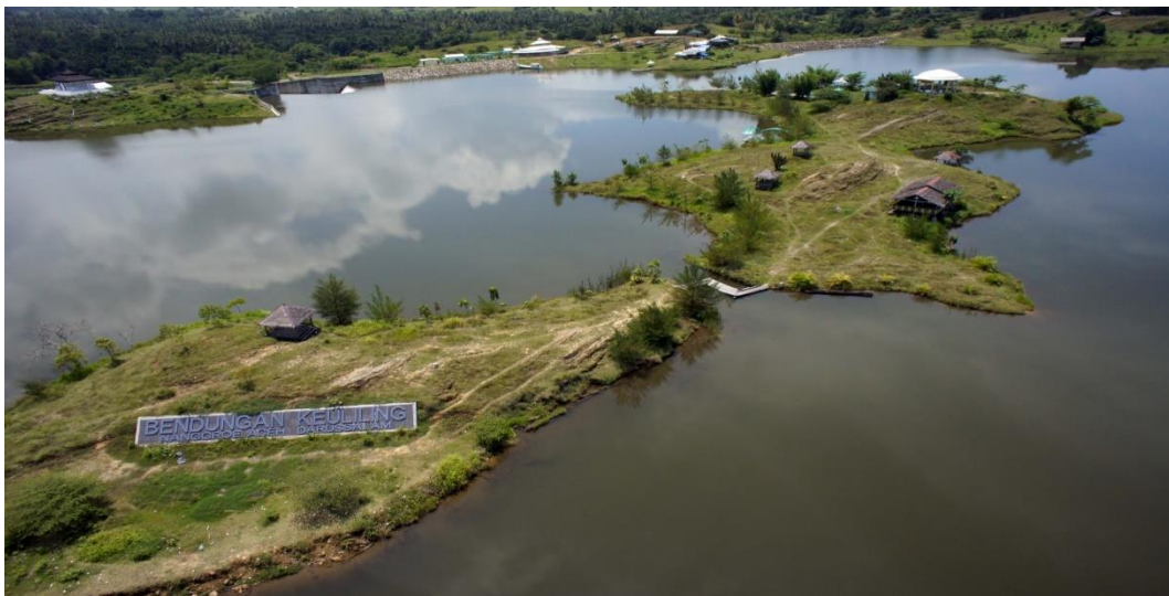
Fig. 1. Keuliling Reservoir as the First Dam in Aceh Province, Indonesia
