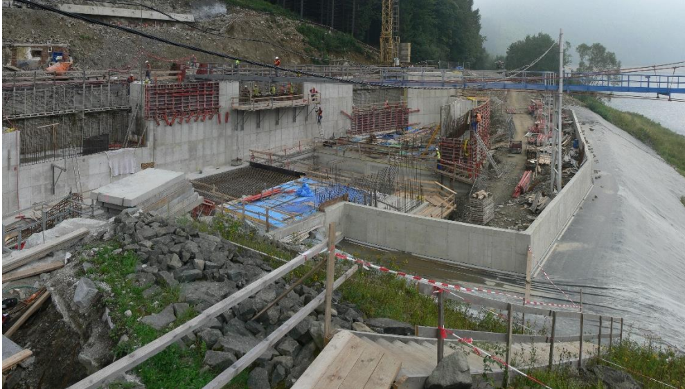
Fig. 5 Concrete cofferdam at the reconstructed dam Šance
