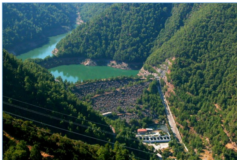
Fig. 3. A general view from Balcova dam.
