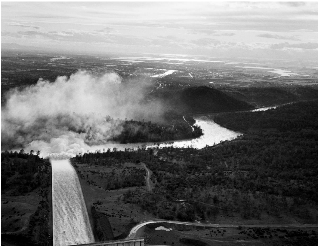
Fig. 3 Photograph of FCO Spillway chute during release of 4248 m 3 /s (February 21, 1986)
