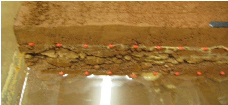
Figure 20: Damage at upstream, middle to left side, near to abutment
