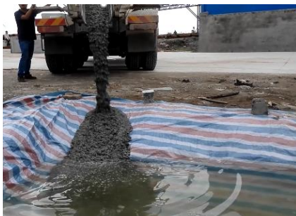
(a) commencement of pouring
