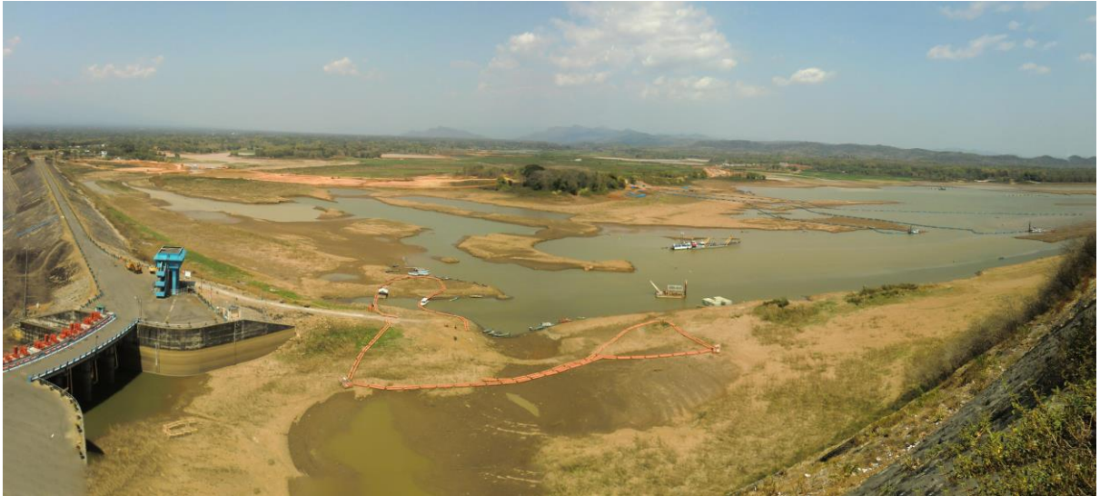
Figure 3. Heavy Siltation requires continues dredging, Source: Nippon Koei staff photo
