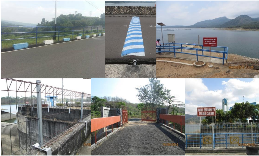
Fig. 5 Security Fences around Main Dams
