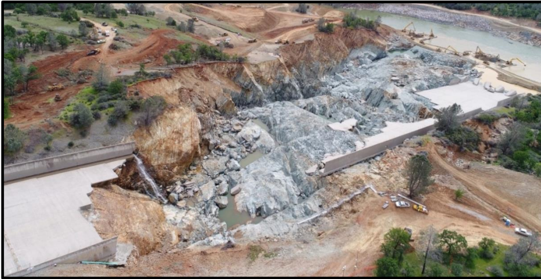
Fig. 3 Aerial view of heavily damaged FCO Spillway lower chute (March 2017)
