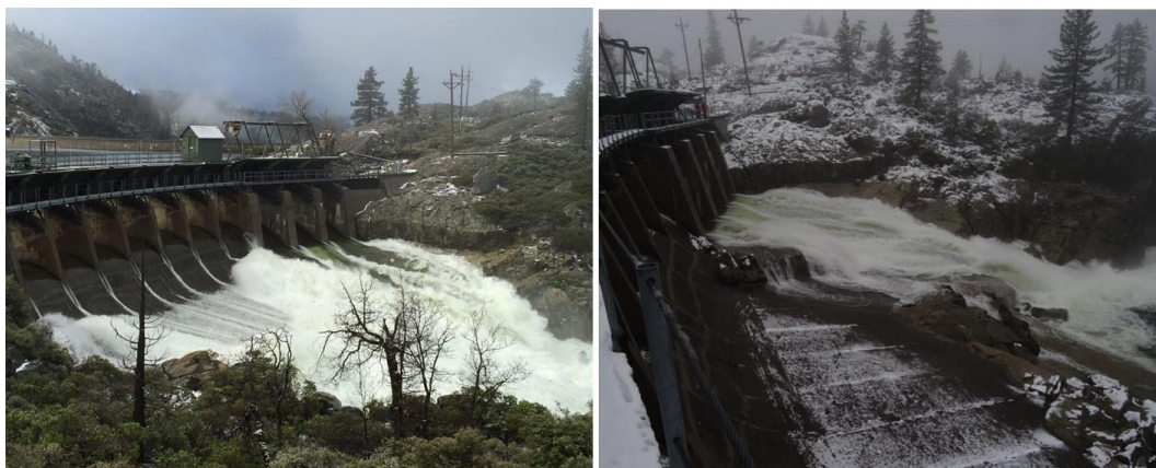
Fig. 6 Discharge on March 6, 8 am (125 m 3 /s (left), March 12, 10 am (30 m 3 /s) (right).
