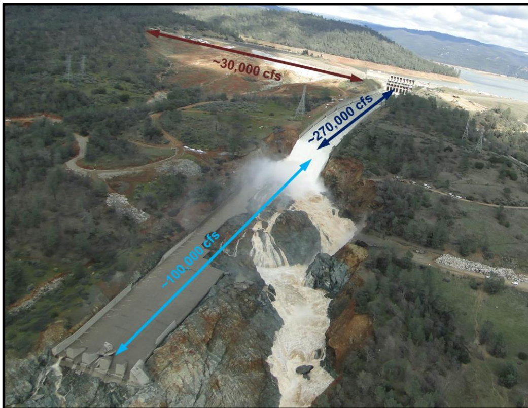
Fig. 2 2017 Oroville Spillway Recovery design objectives projected onto an aerial view of the damaged spillways at Oroville Dam
