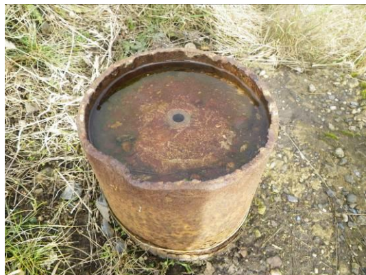
Fig. 6: Lateral and vertical movement monitoring point
