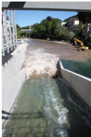
Fig. 7 Ejector ramp flow – Waidhofen Power Station
