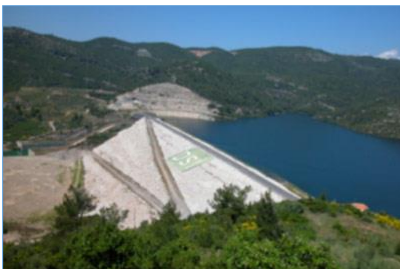
Fig.4. A general view from Tahtali dam
