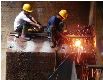
Figure 4.16 Replacing Process of Rail and Brushing Flange Existing
