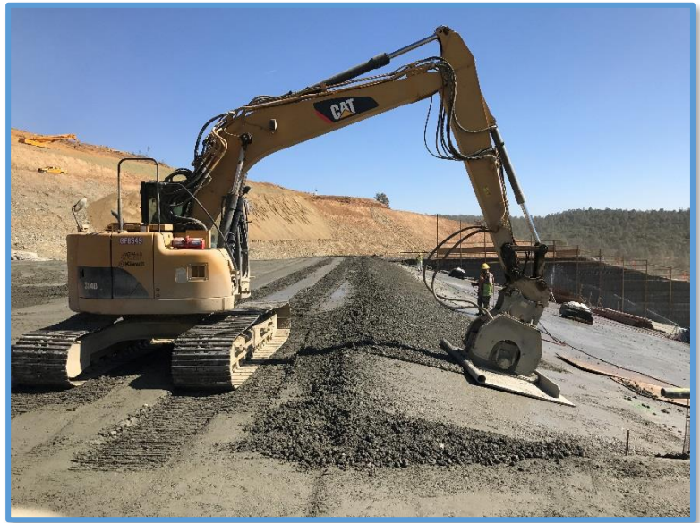
Figure 8- Free Form Construction of 4:1 Slope of RCC
