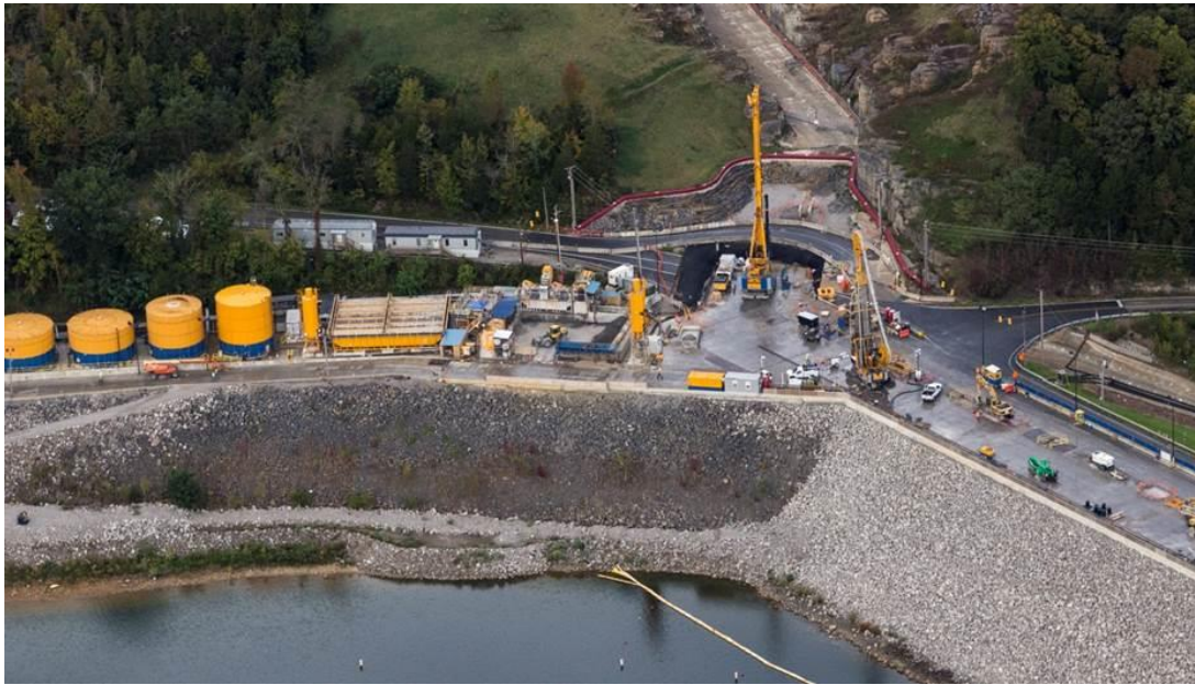
Fig. 1 Site overview 2014 – Slurry Plant, BG 50 Drill-rig and MC128 with BC50 Hydrocutter
