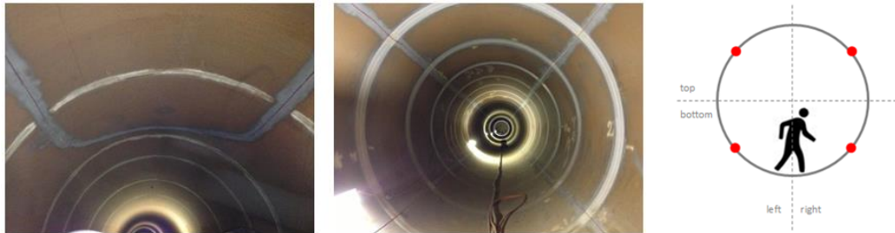
Fig. 10 Strain sensing cable installation inside the penstock
