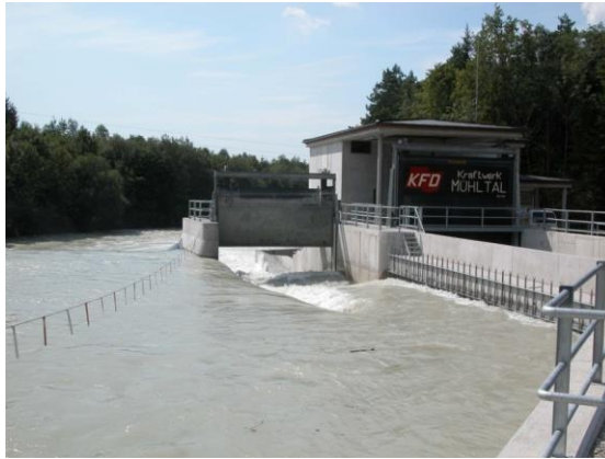
Fig. 17 Fully opened ejector gate – situation at pilot project KW Mühltalwehr / Alm
