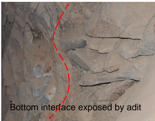
(c) Bedrock and overburden contact interface (d) Bedrock exposed at the slope surface leading age
