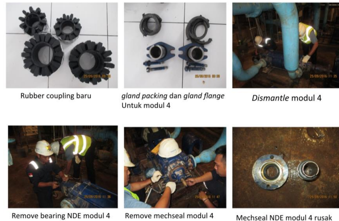
Fig. 5 O&M works in 2016 (BBWS SO documentation)
