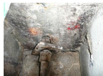
(c) Broken tendon of PS anchor, which was drawn
