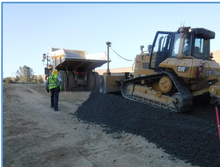
Figure 9 - Test Fill #2 for 4:1 Slope Placement
