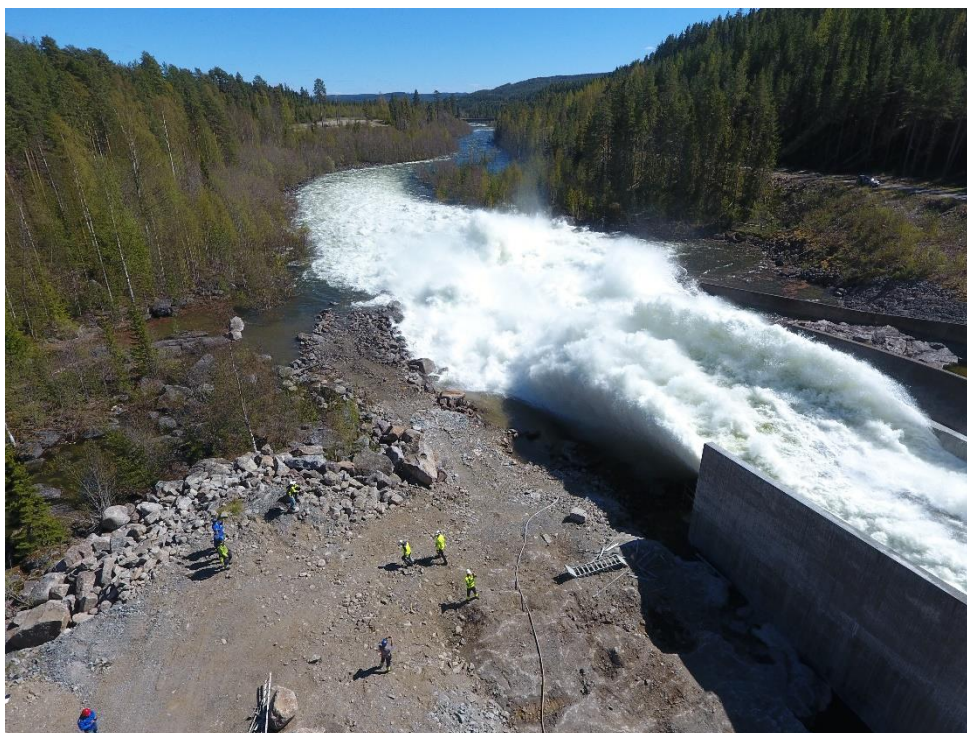
Figure 13: Drone photo from first discharge test, after completed construction (Norconsult, 2016).
