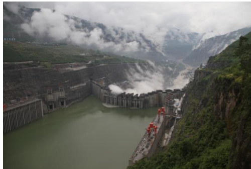
Figure 2. Giant reservoir of the hydropower station in southwest China
