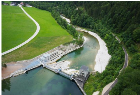
Fig. 30 Aerial photography of ejector plant Gaissulz / Ybbs [3]
