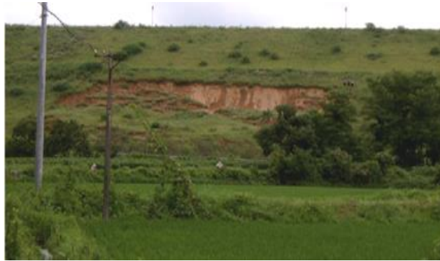
Fig. 3 AG dam incident: downstream slope-sliding (2003)
