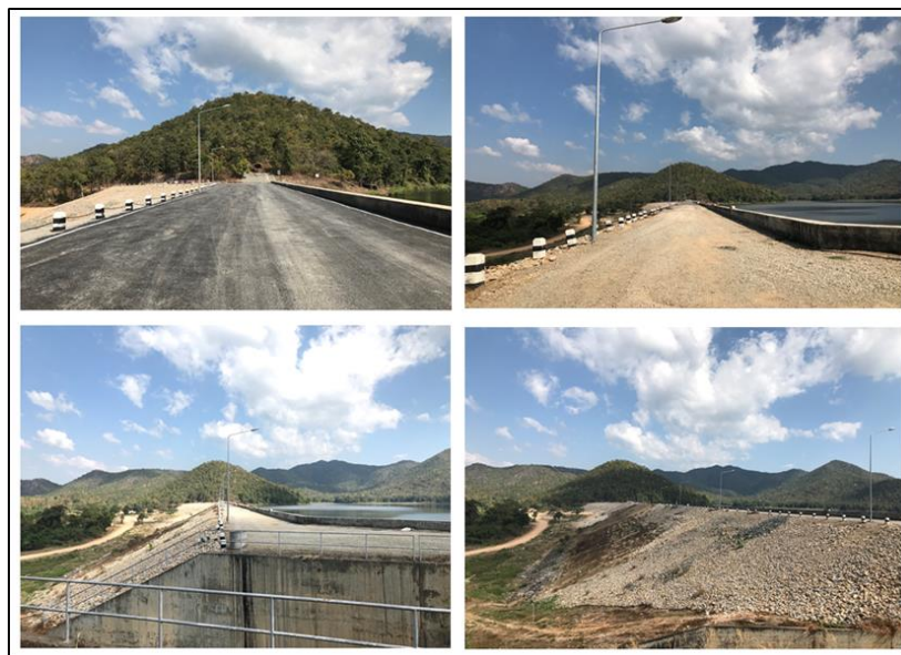
Fig. 10 Mae Thi Dam after completion of Ground Improvement
