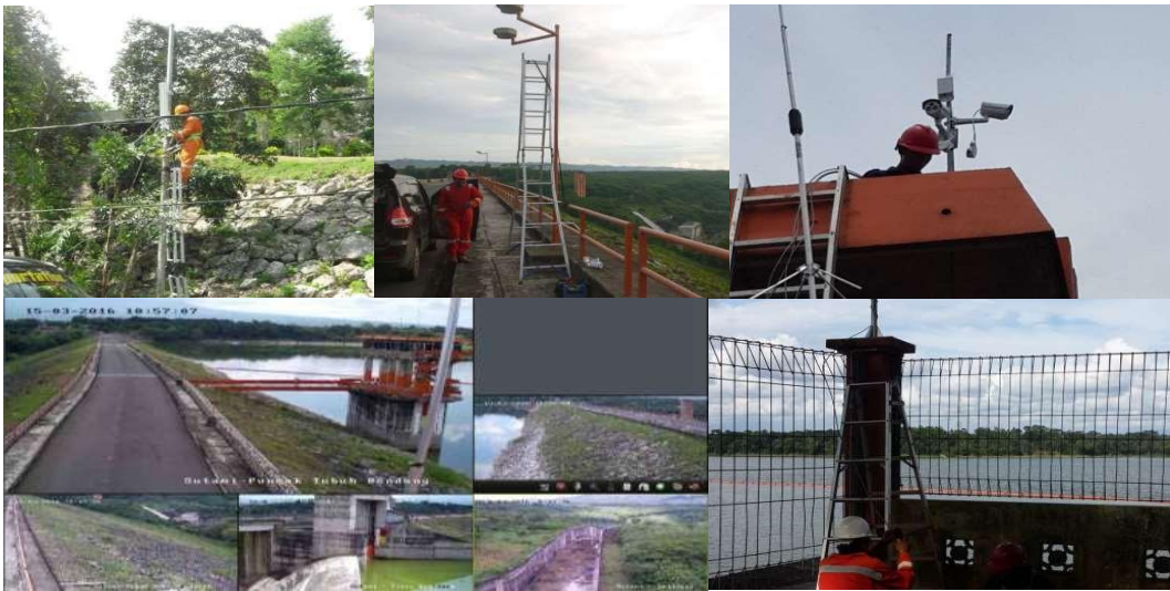
Fig. 3 CCTV Installation
