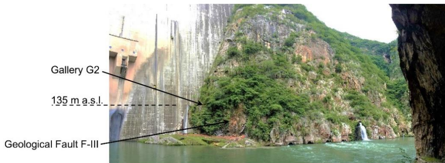
Fig. 1 Panoramic View, left abutment
