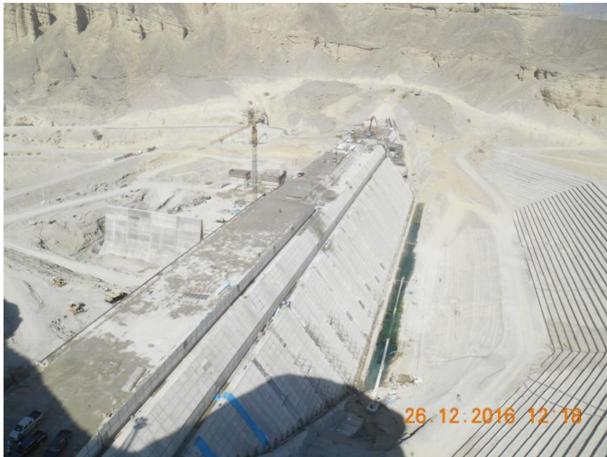
Fig. 4 Berms of Elev.+42 & +50, Dam U/S View
