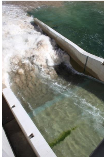
Fig. 6 Waidhofen Power Station: ejector flow at the end of the ejector ramp (mixing zone)
