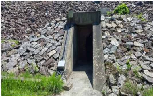
Fig. 3 Appearance of Seepage Measuring Room
