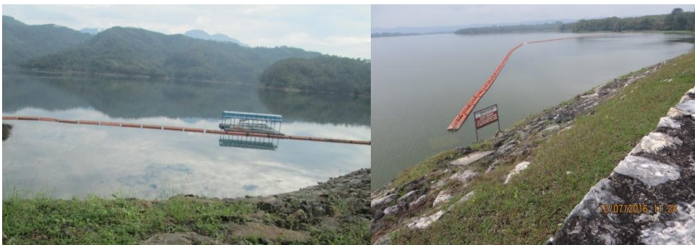
Fig. 6 Trash boom around hydropower intakes
