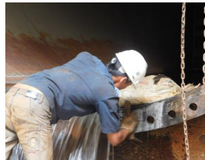
Figure 4.16 Replacing Process of Rail and Brushing Flange Existing
