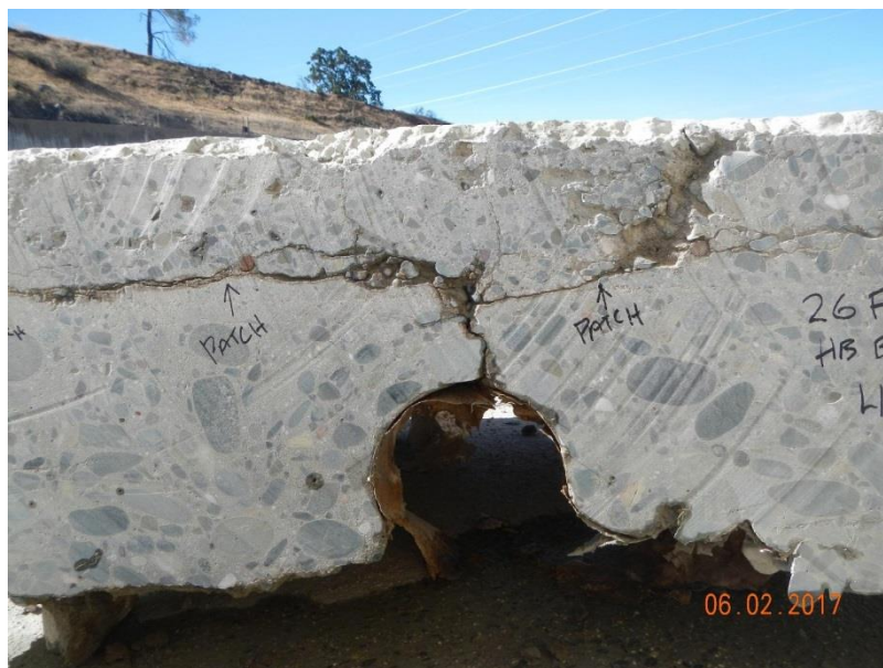
Fig. 8 Section of service spillway chute slab removed during post-incident forensic investigation
