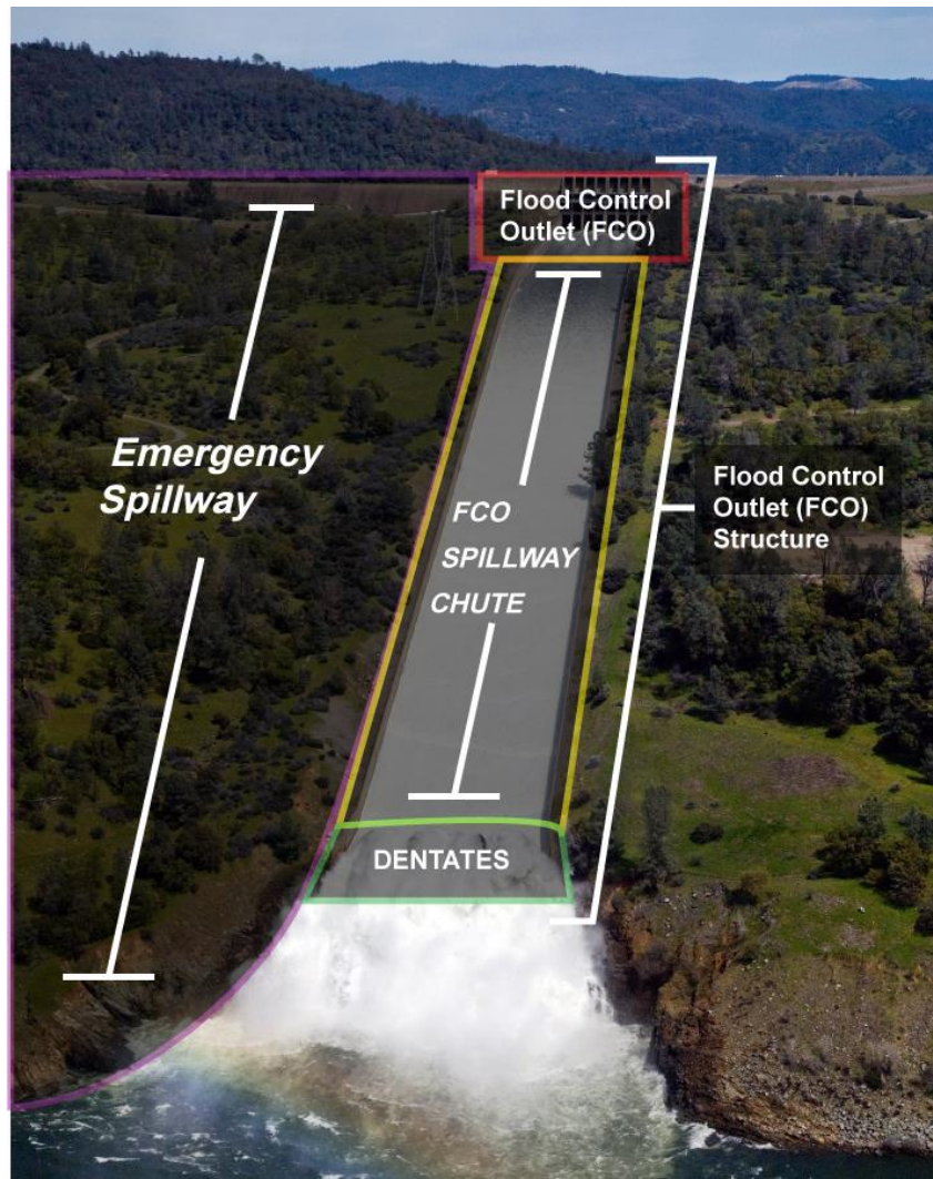
Fig. 1 Flood Control Outlet (FCO) Structure and Emergency Spillway, March 2011
