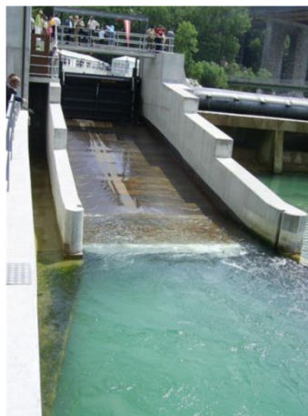
Fig. 20 Ejector ramp – KW Mühlthalwehr/Alm with steel covering
