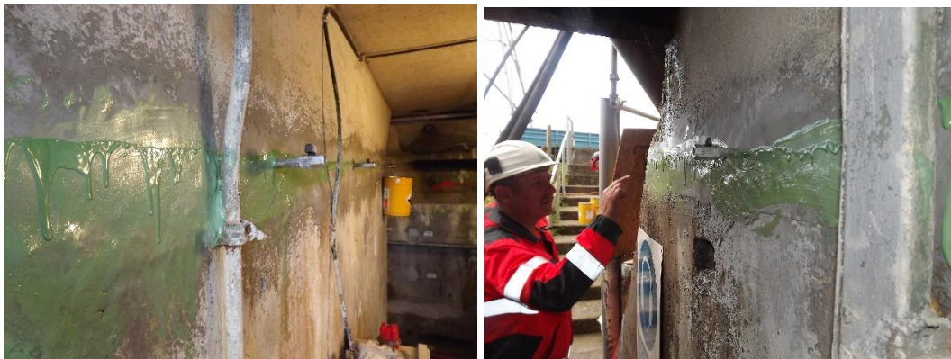
Figure 11: Grouting of the "Dry Cracks"
