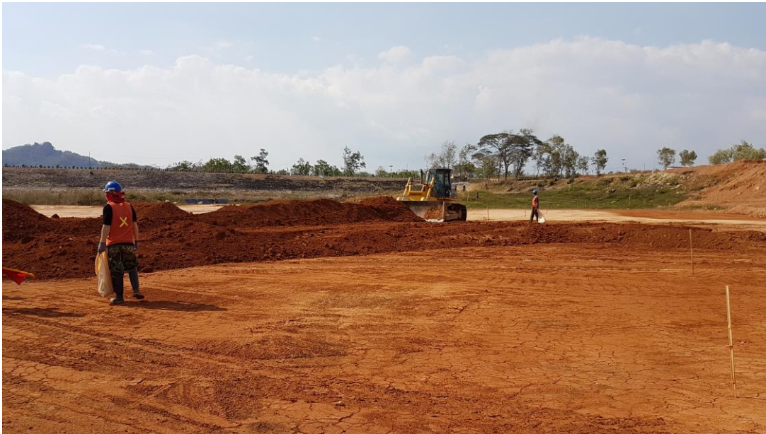
Figure 11. Primary Embankment Spreading. Source: Nippon Koei Staff Photo
