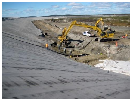
Fig. 9. Bloom Lake, anchorage at the toe of the dam
