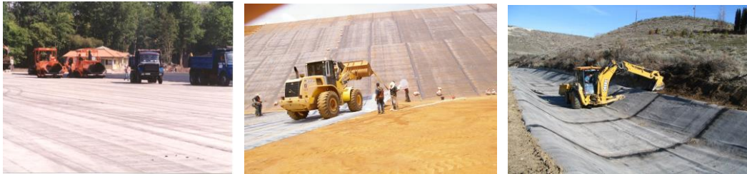
Fig. 3. Tire mounted equipment traffic on top of the BGM
