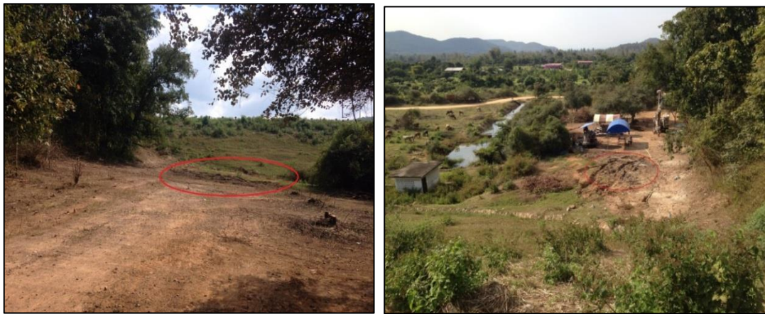
Fig.2 Area of Water Leakage
