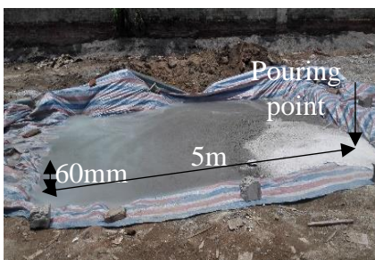
(c) pouring finished
