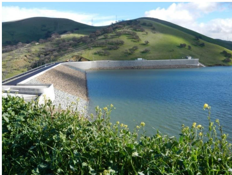
Fig. 6 Completed Los Vaqueros Dam Expansion
