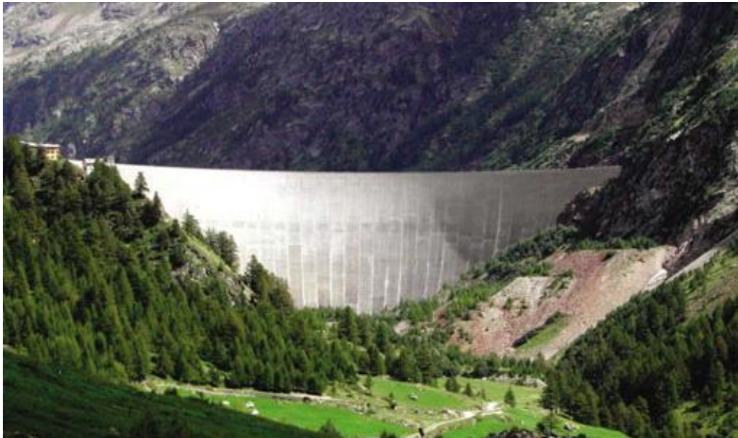
Fig. 1 Downstream view of the dam of Place Moulin
