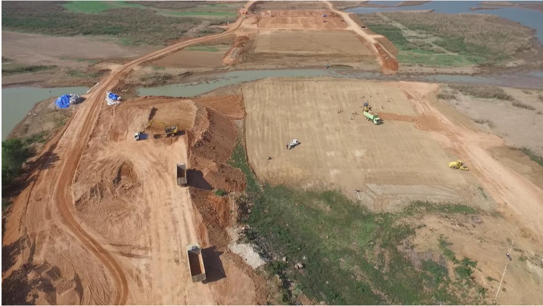
Figure 10. Primary Embankment Placement, Source : Hazama Ando-Wika JO Drone Photo
