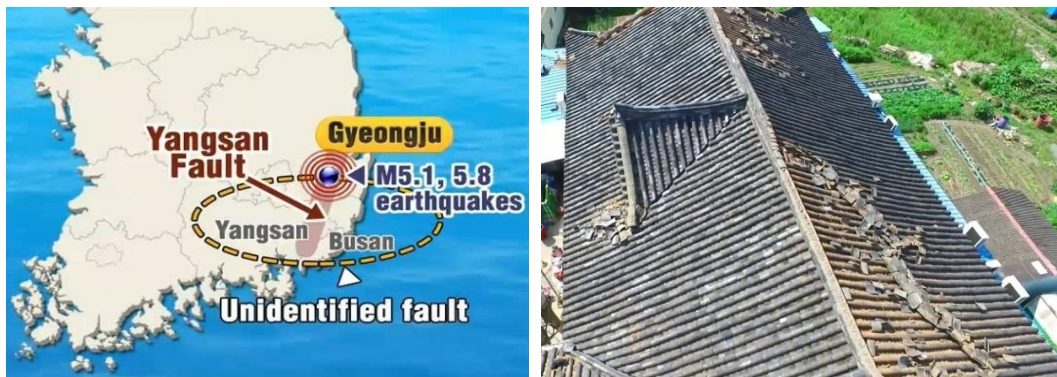
Figure 1. Epicenters and Damage due to earthquake (Source : www.arirang.com & www.ytn.co.kr)
