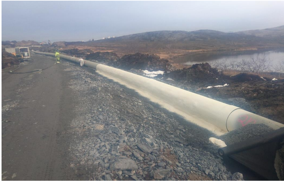
Fig. 1 PU-foam used as backfill
