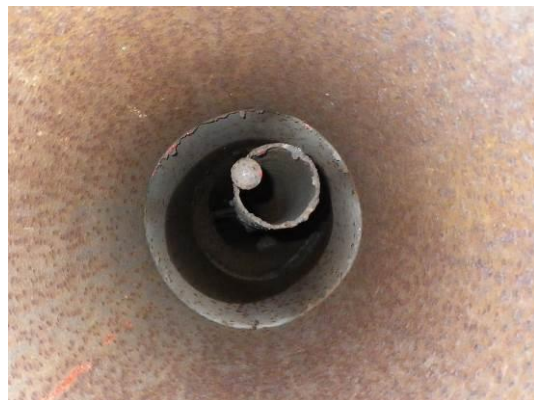
Fig. 4: View into the levelling well
