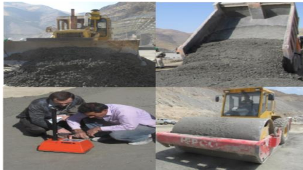
Fig. 5 RCC construction and density testing (Javeh Dam-Iran)
