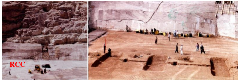
Fig. 3. A) Interface of RCC and clay core; Excavated installation banks [Ref. 3]
