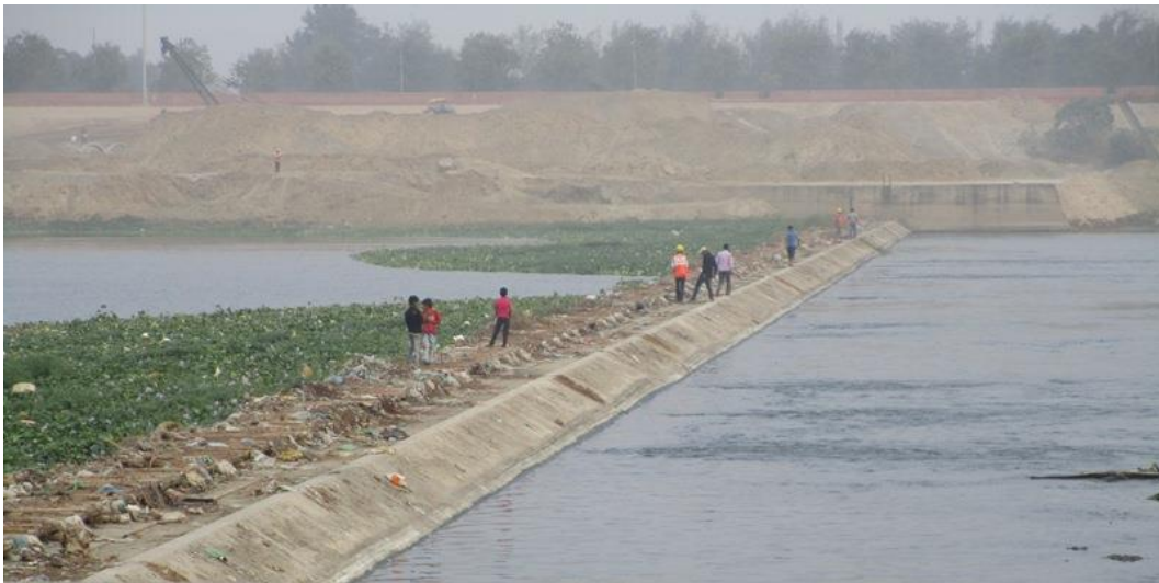
Fig. 2 View to the Gomti Weir in year 2015 before upgradation
