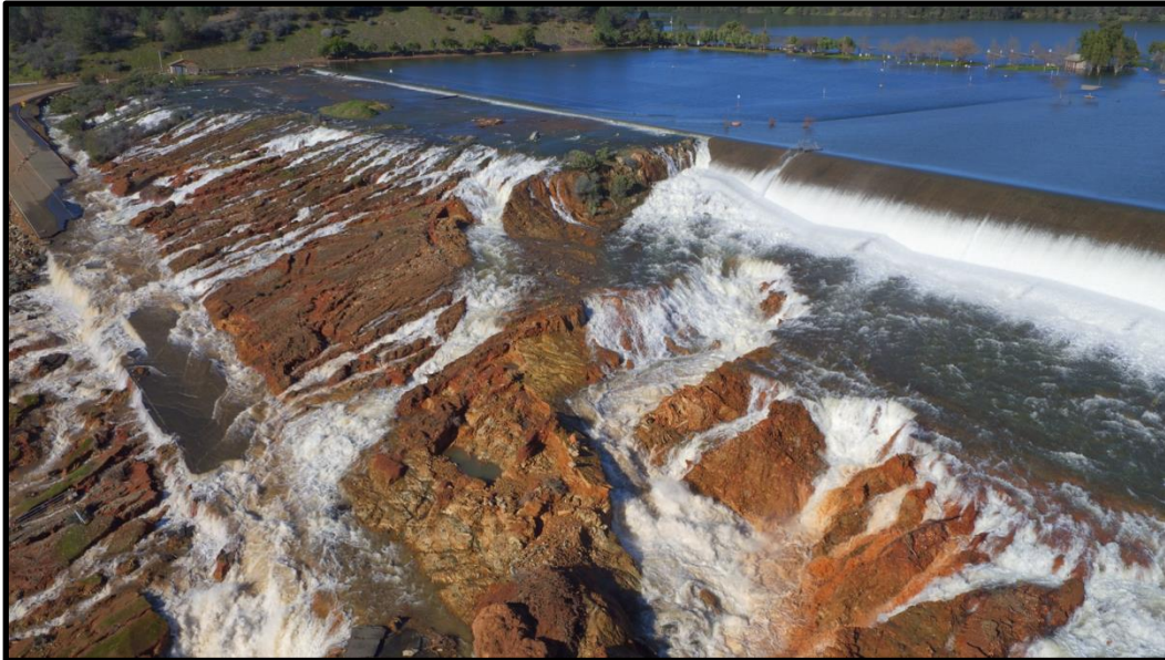
Fig. 6 Aerial view of head-cutting erosion threatening the Emergency Spillway monoliths/weirs during the Feb. 12, 2017 spillway releases
