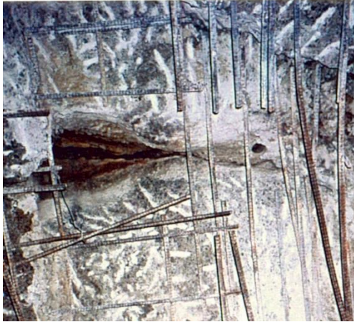
a) eroded crack in TBr above concrete in crown of Block 342
