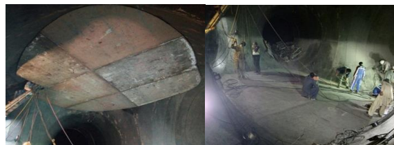
Fig. 17 Photographs of installing deflection plate
