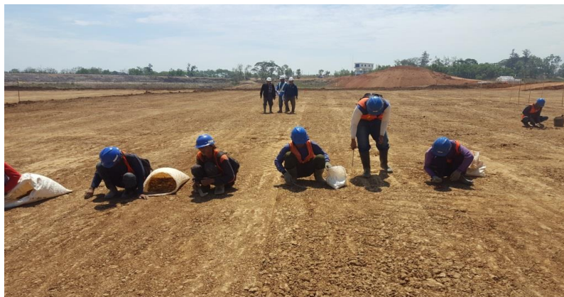
Figure 9. Final inspection of grubbing after stripping and initial compaction
