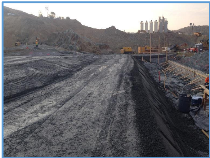
Figure 7 Unformed 1:1 Slope of RCC Structure
