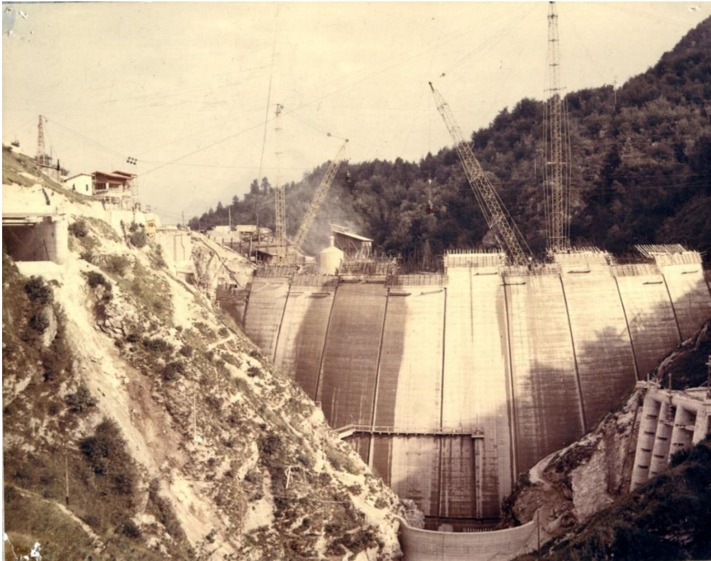
Fig. 3 Ambiesta dam (during construction) Ambiesta barrage (pendant la construction)
