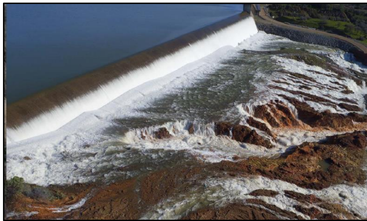
Fig. 11 Emergency spillway headcutting on February 12
