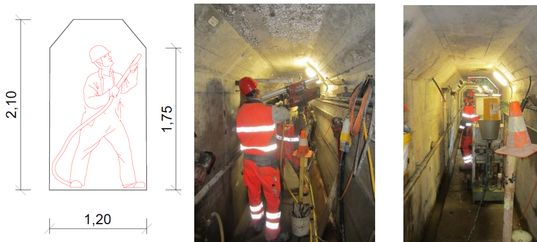
Figure 5: Drilling Works from Inspection Gallery (Hilti DD200)
