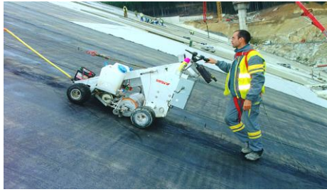
Fig. 4. Ultrasound equipment to test BGM welds
