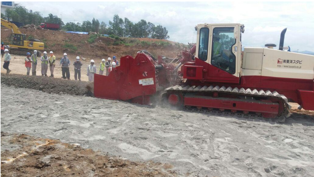
Figure 13. Stabilizer Machine mixing soil cement. Source: Nippon Koei Staff Photo
