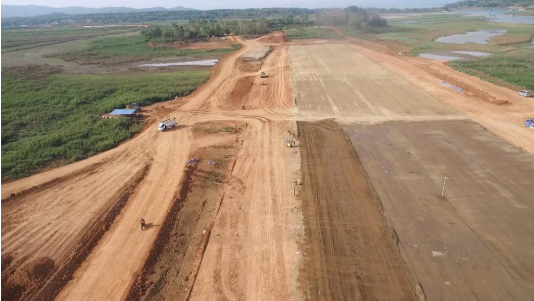
Figure 14. Soil Cement Placement on Primary Embankment. Source :Hazama Ando-Wika JO Drone
