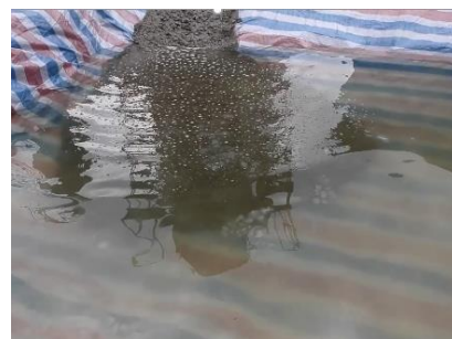
(b) process of pouring
