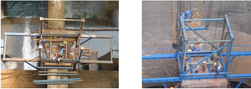
Figure 4.6 Installation Lifting Table Component
