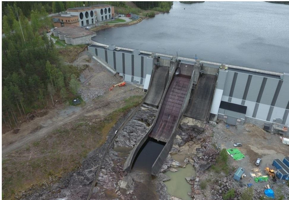
Figure 3: Aerial photo of Ramsele dam and spillway (Norconsult, 2015).
