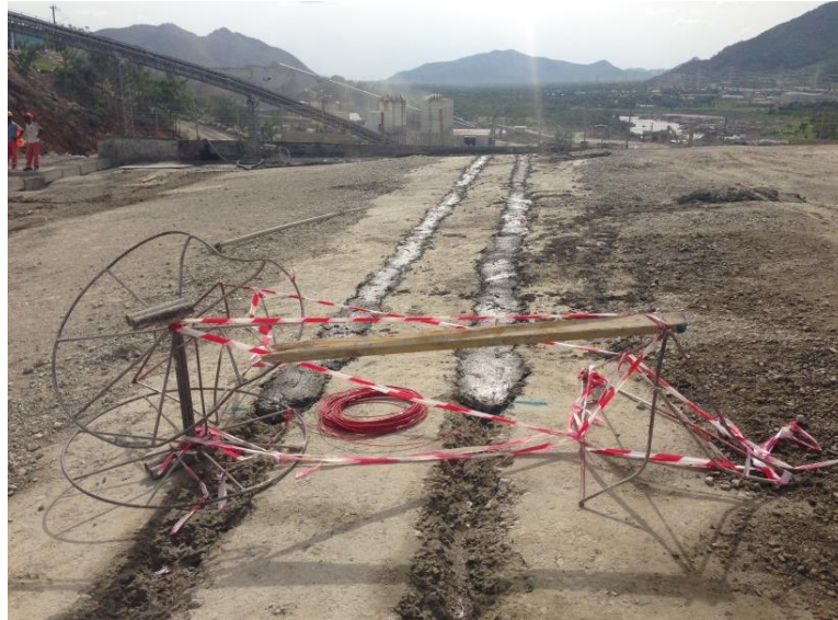
Fig. 3 Sensing cable installation at Grand Ethiopian Renaissance Dam (GERD)
