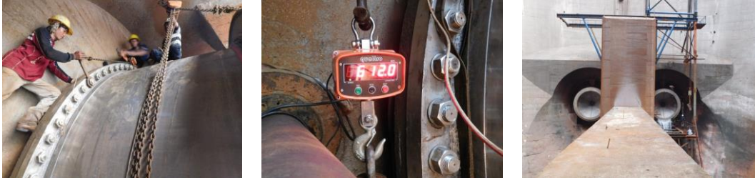
Figure 4.17 Bolt Installation Process with Specified Load
