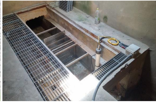
Fig. 4 Inside Seepage Measuring Room
