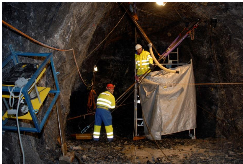
Fig. 3 Installation of dilatometer system in small exploration gallery
