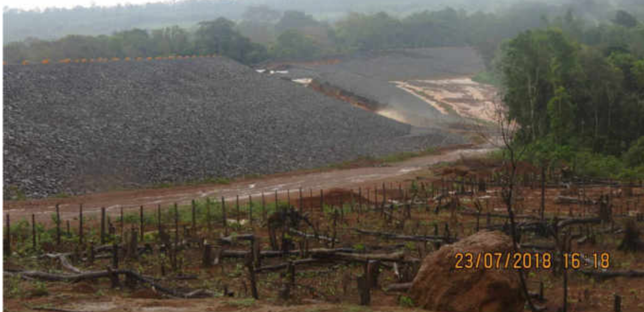
Foundation on subsoil Grouting - Consolidation
