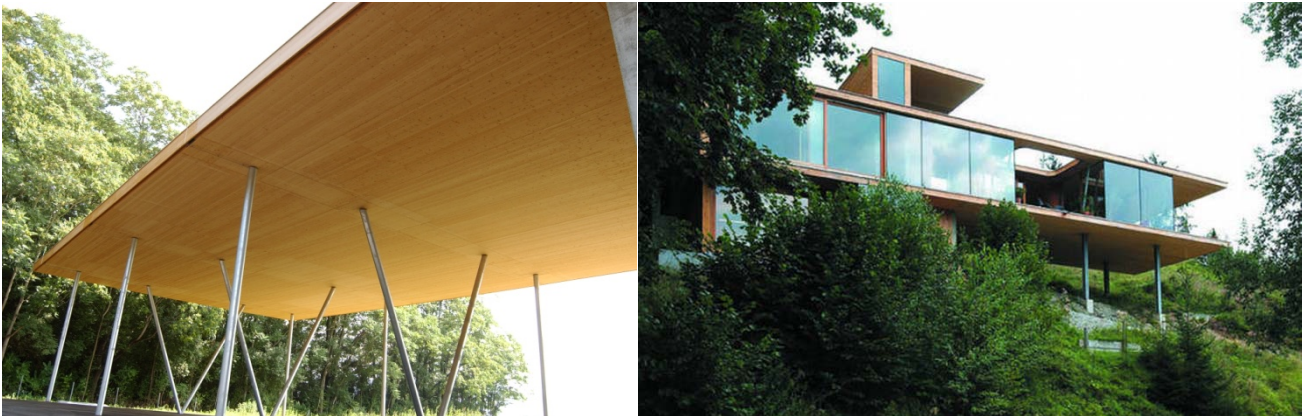
Figure 1.1. examples for CLT plates with column support.
