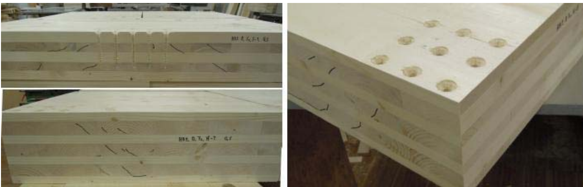
Figure 5.2. observed typical failures in test configuration 1
