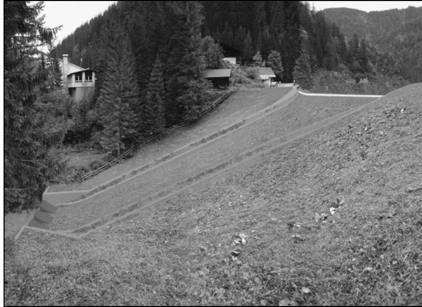
Figure 11. Overflow Spillway after Revegetation of Chute and Stilling Basin
