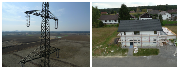
Figure 1. Two examples for wiry structures. The left image shows a power pylon and the right image a scaffold in front of a house.
