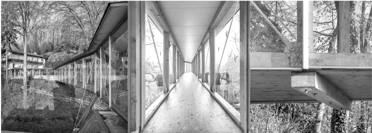
Fig. 5 Impressions of the timber footbridge 'Building Corridor Bad Gleichenberg'
