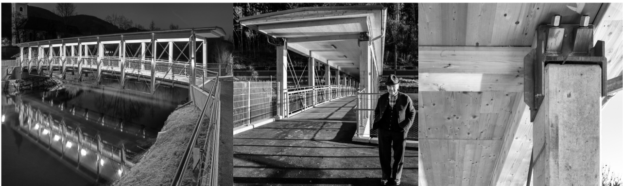
Fig. 9 Impressions of the timber footbridge 'Truss Bridge Kindberg'
