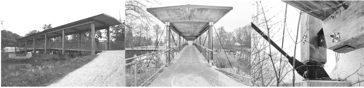
Fig. 3 Impressions of the timber footbridge 'Leonardo Bridge'
