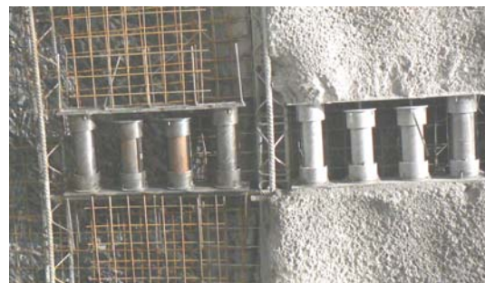
Figure 2. Yielding elements of the type LSC integrated in a shotcrete lining at the Tauerntunnel. Photo: Vergeiner
