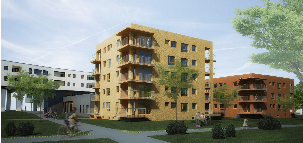
Fig. 25 image of a five storey residential building of the project “Peter Roseggerstraße“[22]
