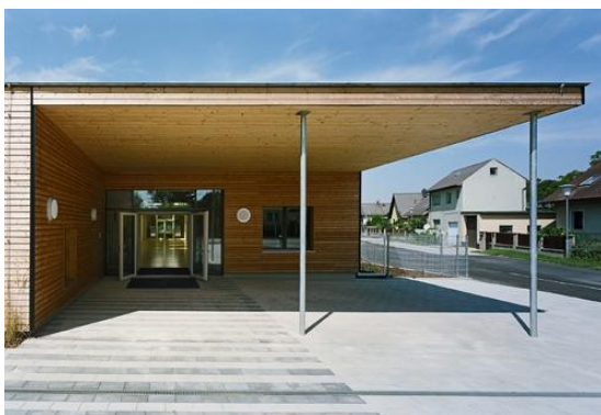
Figure 1: Solid timber building system with CLT, partially supported with columns
