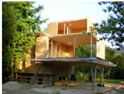
Figure 1: Solid timber building system with CLT, partially supported with columns
