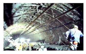
Fig 12. Three rows of yielding elements installed in the shotcrete lining at the Semmering base tunnel
