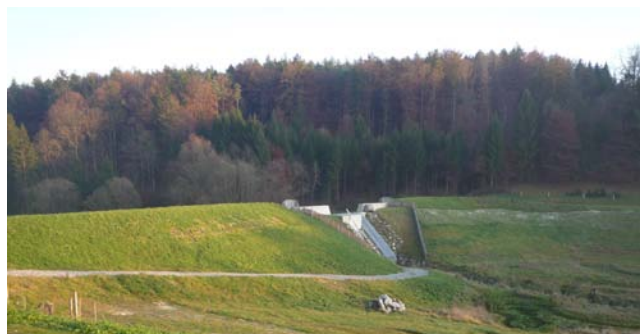
Figure 7: Retention Basin Labuch
