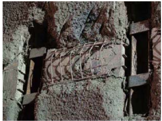
Figure 8. HiDCon element installed in shotcrete lining (from [12])
