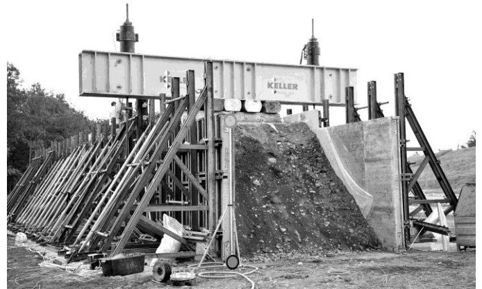
Figure 1. Experimental dam in the vicinity of the hydroelectric power plant
