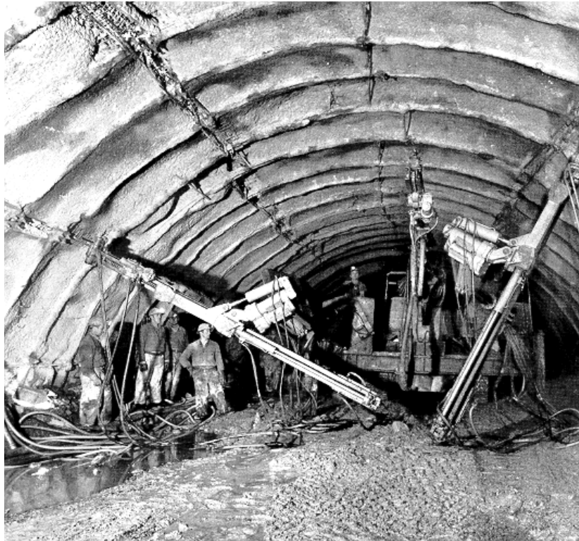
Figure 1: “Tauerntunnel” / Austria; Shotcrete lining with deformation gaps [4]
