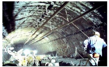
Figure 3. Application of a ductile lining system using Lining Stress Controllers (LSC) at the Semmering basis tunnel
