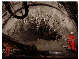
Figure 2. Failure of stiff lining at the Gotthard basis tunnel due to excessive deformation of the rock mass
