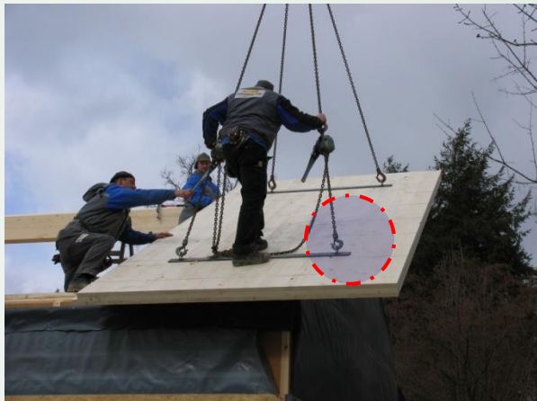
assembling of roof elements
