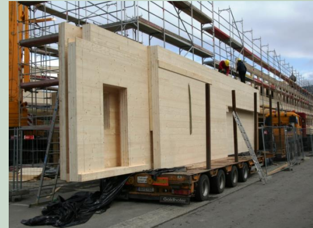
discharging (building site)
