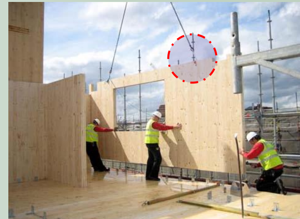
assembling of wall elements
