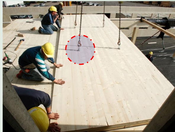
assembling of ceiling elements
