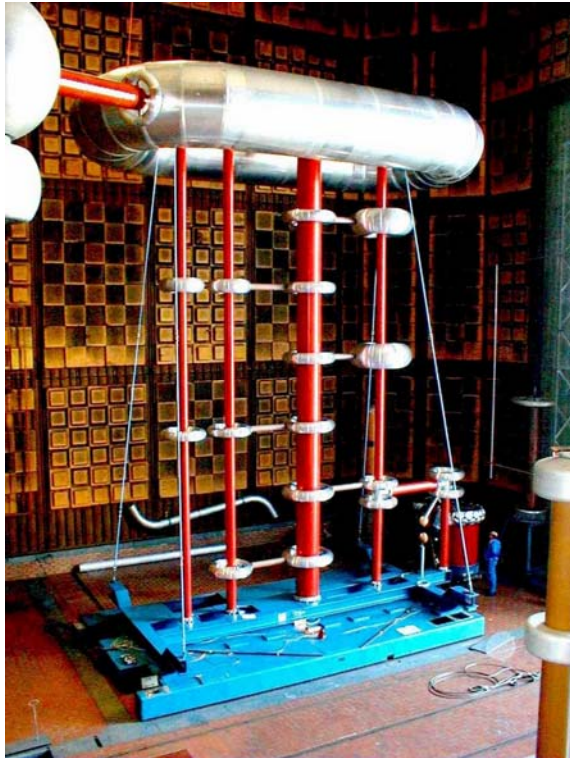
Fig. 18 DC generator for 1200 kV output voltage (Manufacturer: HIGHVOLT Dresden GmbH)
