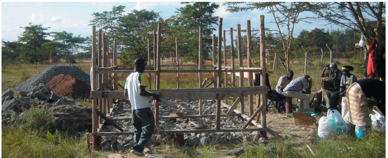
Fig. 3 JENGA design-build construction site at JKUAT, Nairobi
