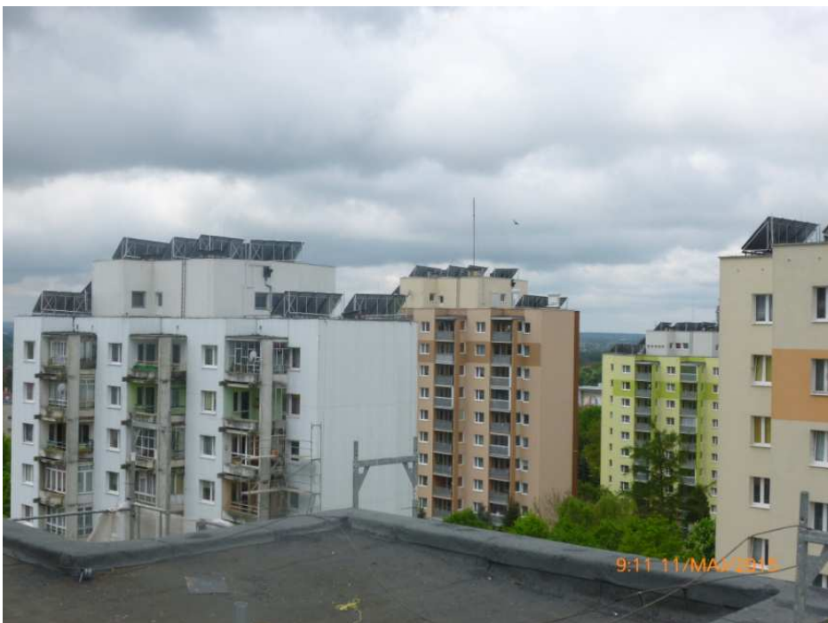
Fig. 2. Collectors on the roofs of high rised buildings arranged in two levels - making the most of limited roof area (photo: A. Ostanska)
