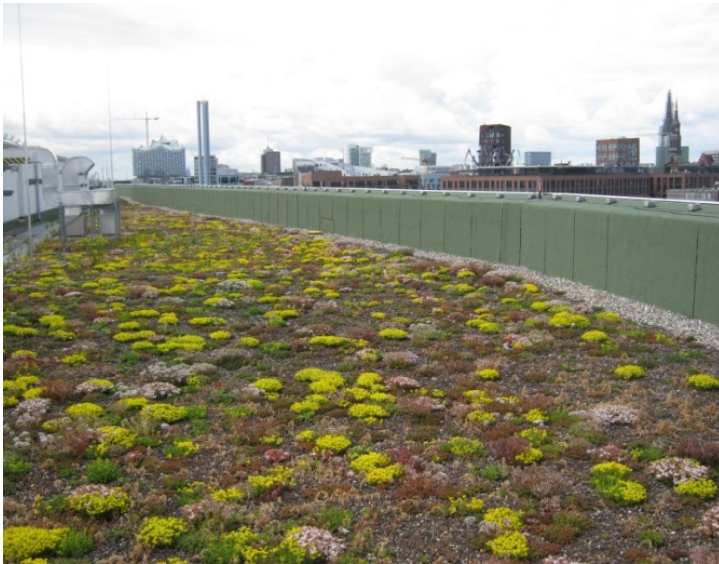
Fig. 2 View over the HCU green roof
