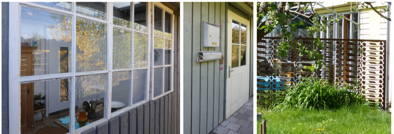
Fig. 11 as one example, the 'nordern corridor' was built with windows and doors of demolished buildings, giving the entrance area 'second hand aesthetics'. Industrial waste like laser-cut steel plates was transformed into a spatial element (pictures 2015)
