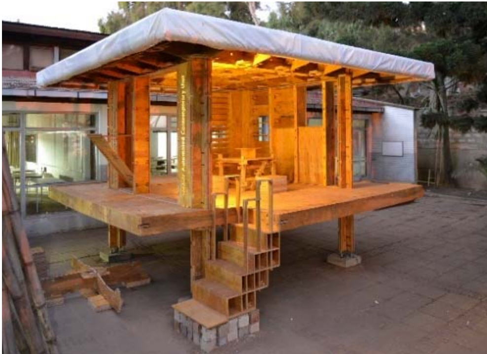
Fig. 3 MACU – half ready construction and the finished one ( assembling time 10h)
