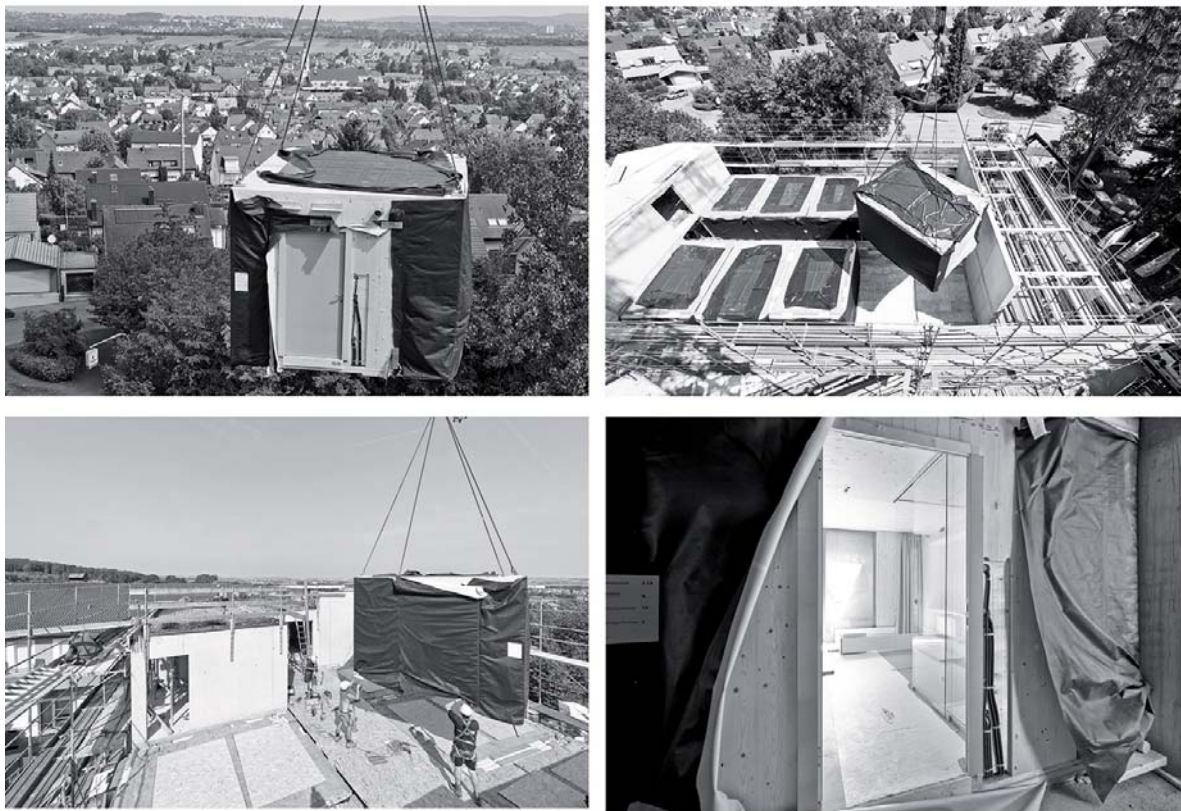
Fig 3 a – d Assembly and Installation Sequences of CLT-Room Modules
