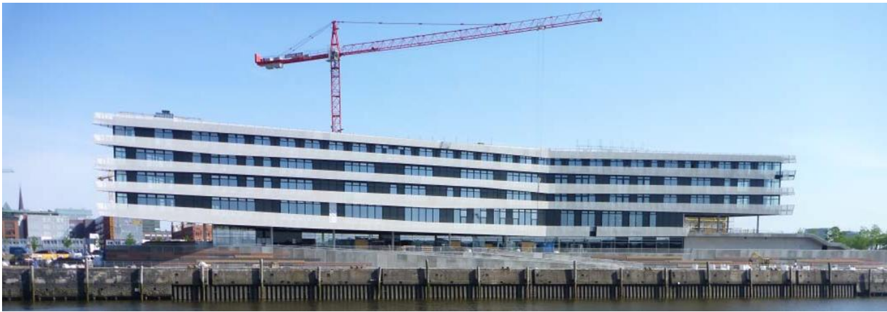
Fig. 3: South view of the campus building HafenCity University, Hamburg
