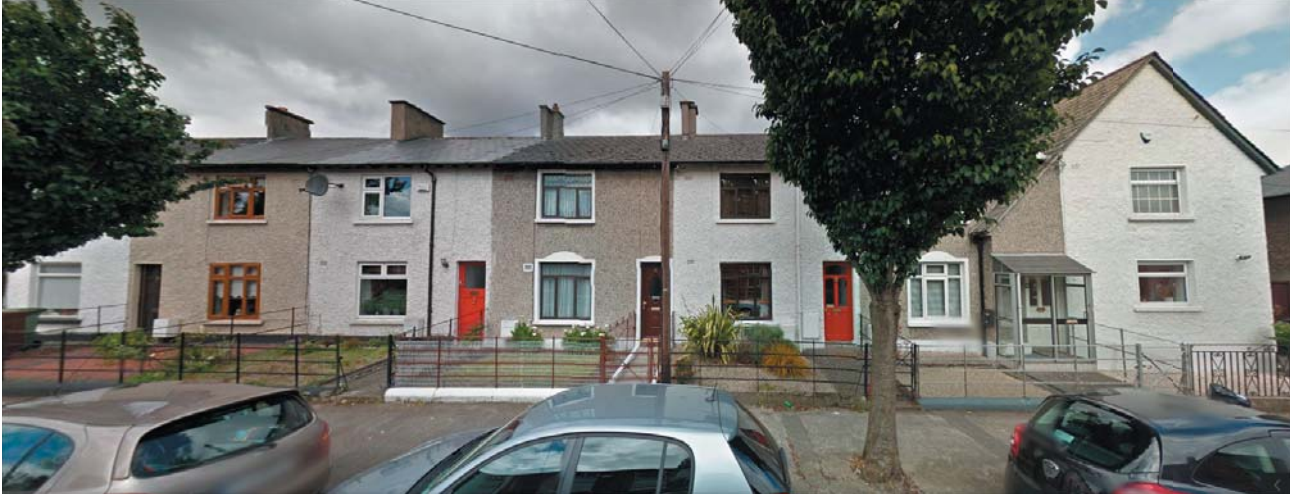
Fig. 1 Row of terraced housing with through wall vents visible on front facades of homes.
