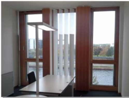
Fig. 7 LED Lighting; Sun Shutter with partly Translucency
