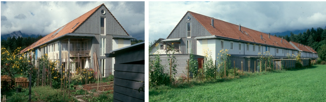
Fig. 2 left: view from East with private gardens and units individually coloured to the south right: view from North-East showing the communal access with the connecting corridor which was designed as a multifunctional space with 261 cm inner width. (Pictures taken 1989)
