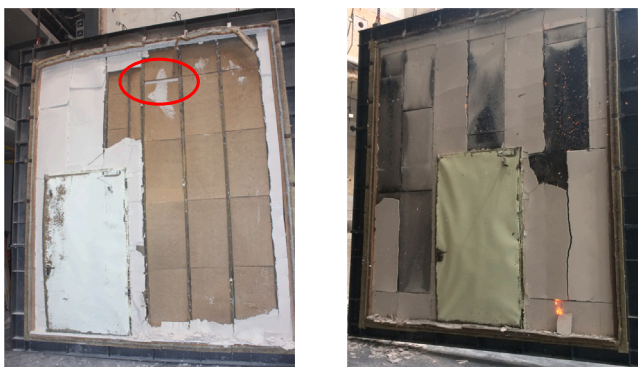
Fig. 30. Failure of gypsum plasterboards when the door is in right position (DR) and the door is in central position (DC). (For interpretation of the references to colour in this figure legend, the reader is referred to the web version of this article.)
